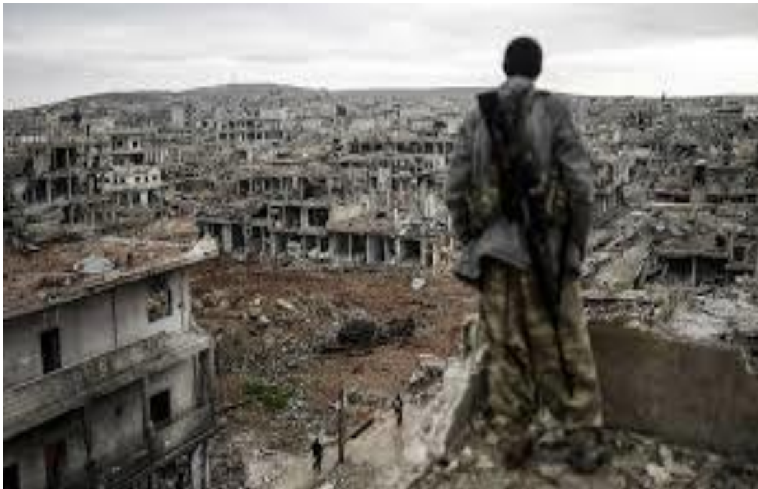
Physical Infrastructure in Disrepair (Syria)
