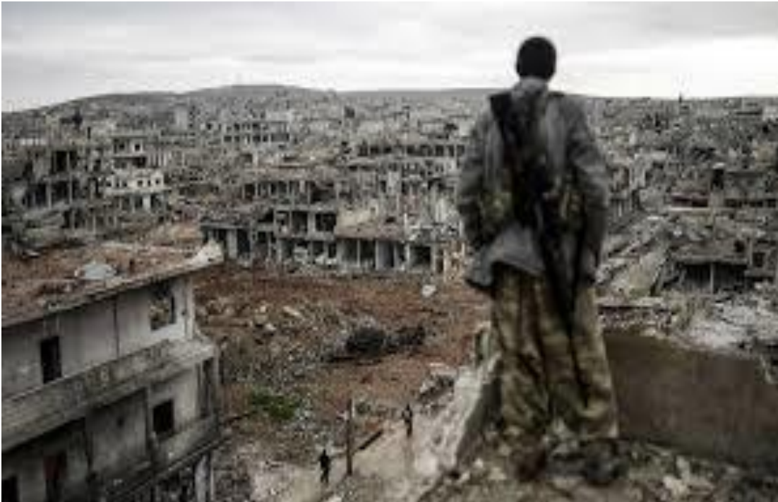
Physical Infrastructure in Disrepair (Syria)
